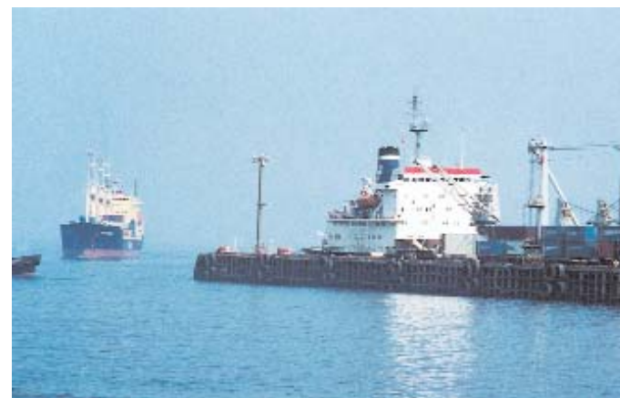
Muelle Industrial SPCC. SPCC Industrial Pier.
